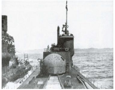
A 1200-hp electric motorgenerator on each shaft drew electricity form her storage batteries to drive her submerged. With a clean bottom this propulsion plant gave her a top speed of 18.7 knots on the surface and 6.5 knots below snorkel depth.
